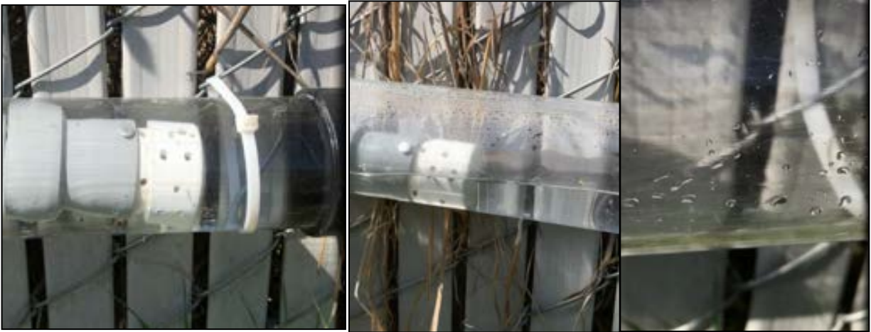
Figure 11 (left-right)—Extraction hose within flooded sewer lateral prop. Water partially extracted from sewer lateral prop. Close-up of sewer lateral prop following extraction with no remaining water, allowing for successful camera inspection.
