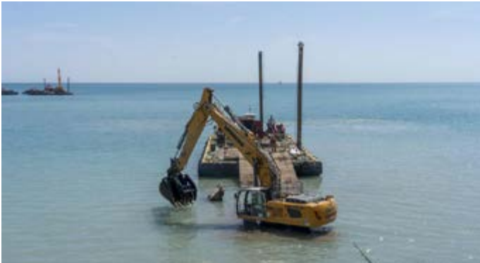
Michels Construction, Inc.
